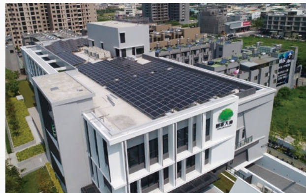
Education Building in Wuri, Taichung: This building has acquired the U.S. LEED Green Building Gold Certificate and has the highest installed capacity of solar panels for self-use in the financial industry (183 kW), generating 234,000 kWh of electricity or reducing 130 tons of carbon emissions each year.
